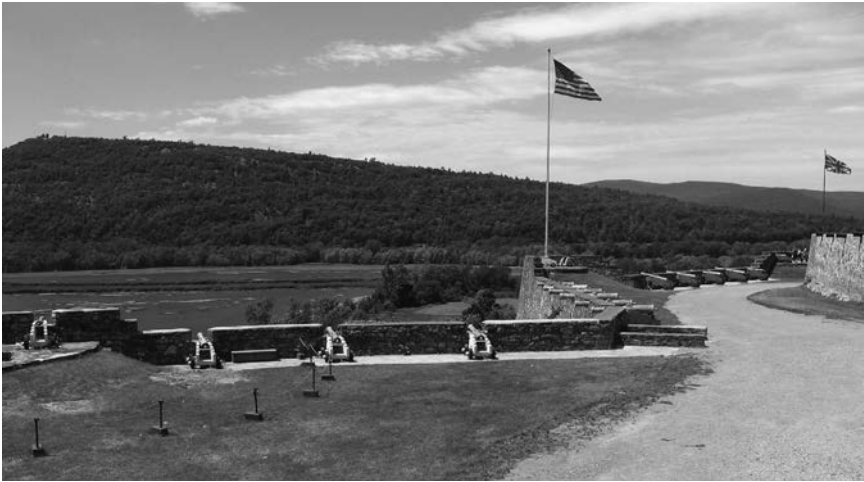
Figure 5.1 The outer wall at Fort Ticonderoga.
